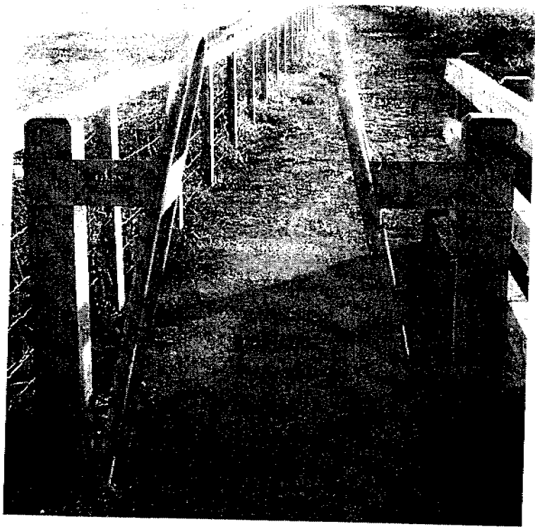
Galvanized steel access control barrier supplied by FEARN (Truck Bodies) Ltd of Rotherham to be installed at bridge entry points. Barriers are 1500mm high, and fixed to 150x150 H/W posts 1200mm high. Gap at base is 1000mm, narrowing to 350mm at top. Designed to permit access by cyclists and wheelchair users but prevent entry by motorcycles and horses
